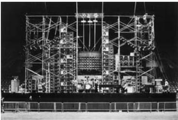
In the United States, especially the band Grateful Dead tried to solve this problem via a gigantic piling up of loudspeakers. The „Wall of Sound“ was developed and optimized by the band's sound engineers for years and it included up to 641 individual loudspeakers with a total RMS power of 26.4 kW. In miniature, a similar concept was adopted by Udo Klempt-Gießing for the cult band Grobschnitt from Hagen, Germany.
